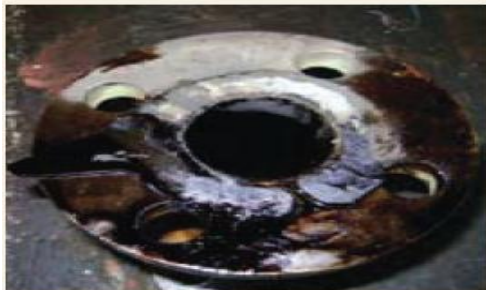
Reused torn gasket that caused the leak at the flange connection
