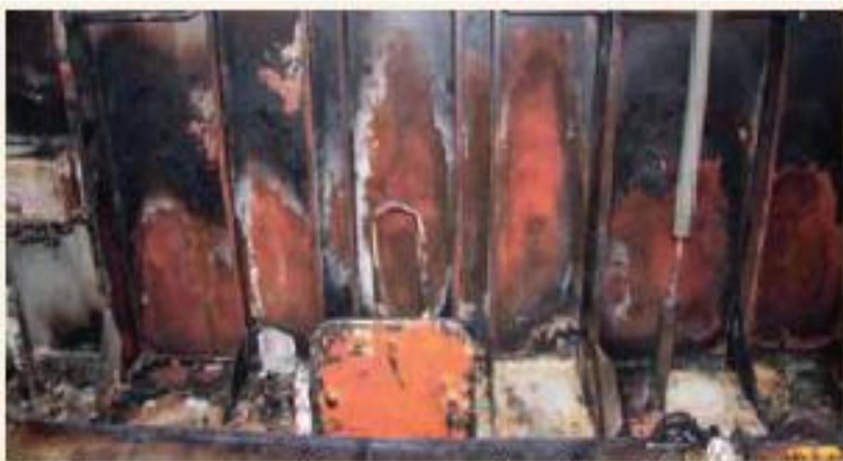
Fire damage to paint and fittings on wavebreaker and deck
