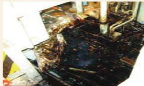
Fuel oil leakage on fuel pump side
