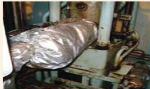
Corrective action implemented – fuel inlet pipe re-connected with new gasket and covered with insulation and containment covering
