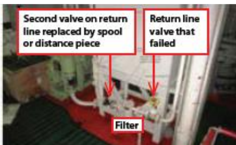
Redundant valve replaced by Spacer Pipe
