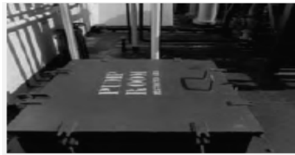
View of pump room hatch in shut position
