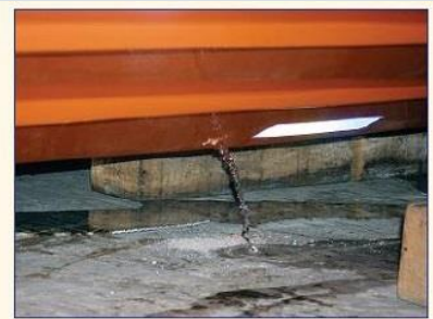
Figure 4: Accumulated water being drained through hole made in outer hull of rescue boat
