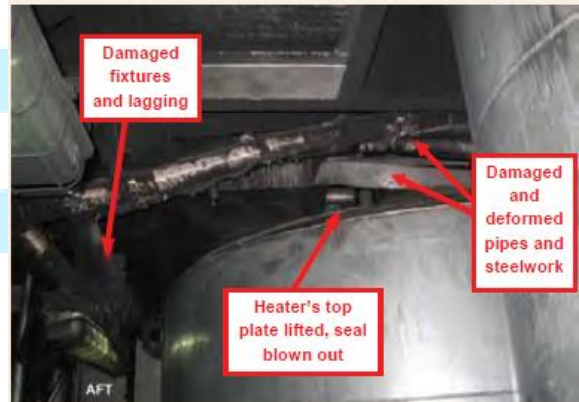
View of damage between top of heater and overlying grating
